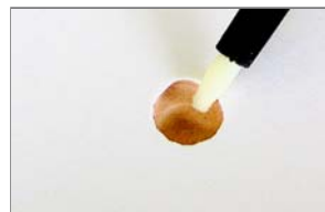
6. Apply StoneLux® Tile Primer in a thin, even coating to all surfaces and allow to evaporate
