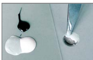
1. Use the Colour materials to create a shade that blends in with the colour of the tile in need to repair; apply the mix-
